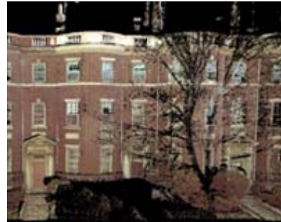
Building Facade Survey
